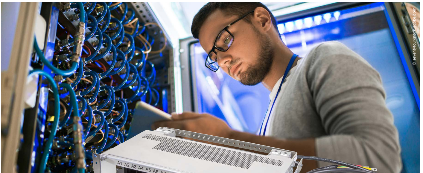
Providing reliable power supply and protection: High Power-D-Box with grounding busbar, 8345 circuit breakers and 3PAR cable set
